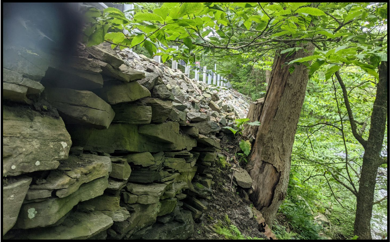
Figure 3: Steep embankment and stone wall photo
